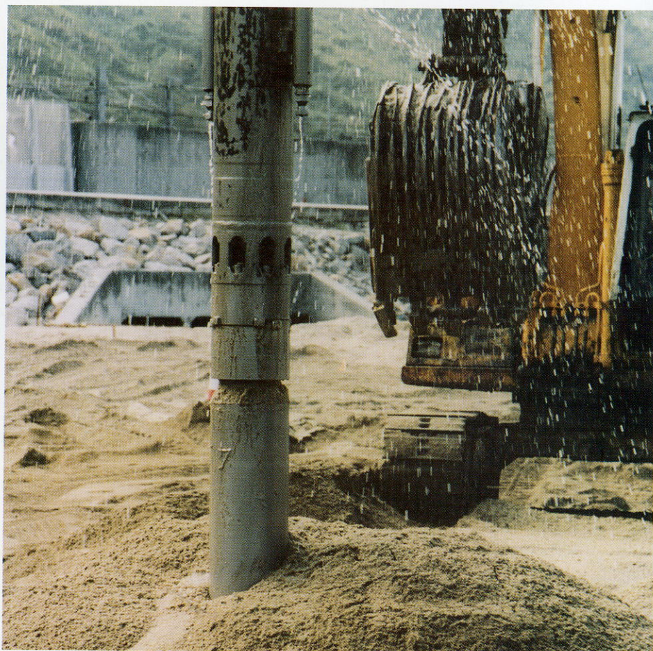
Vibrocompaction of reclamation made of sand, carried out by the 140HL and supported by lateral water jets.
