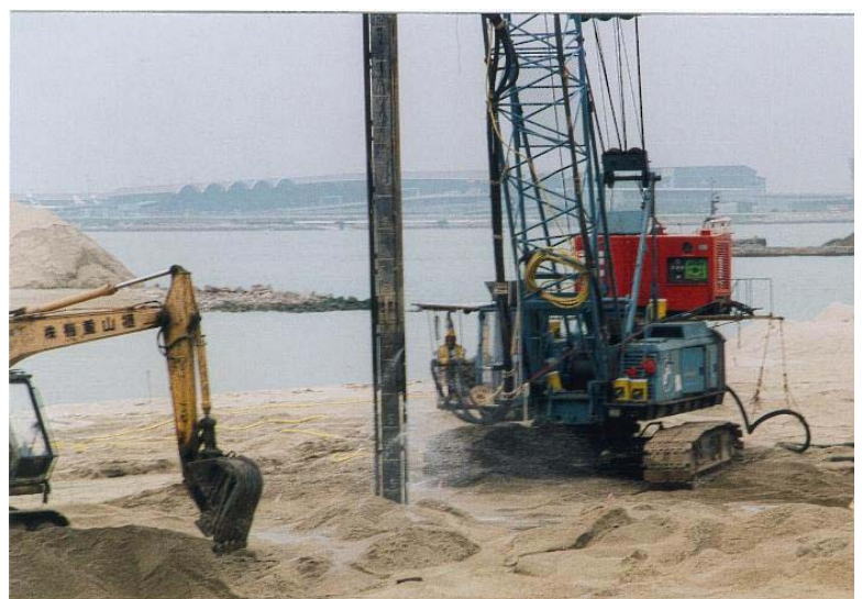
140HR Vibrolance for vibro-compaction of 25m deep on a regular grid, in Hong Kong
