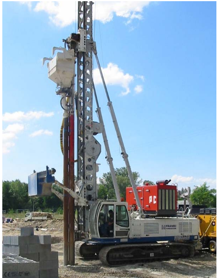
140HR Vibrolance with BFS (Bottom Feed System) mounted on a rig driving 6m deep stone columns, in France
