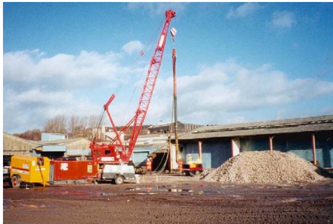
160HR Vibrolance for vibro-replacement by stone columns in Stoke on Trent, in England
