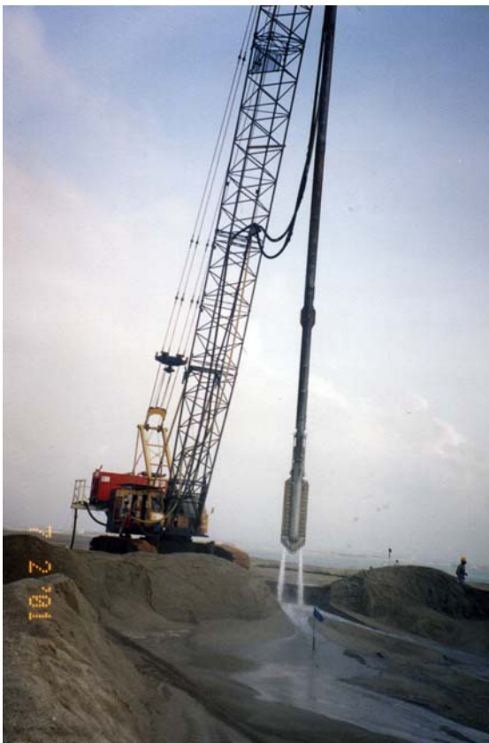
400HR Vibrolance with water jetting for vibro-compaction of 25 m deep on a triangular grid, in Singapore
